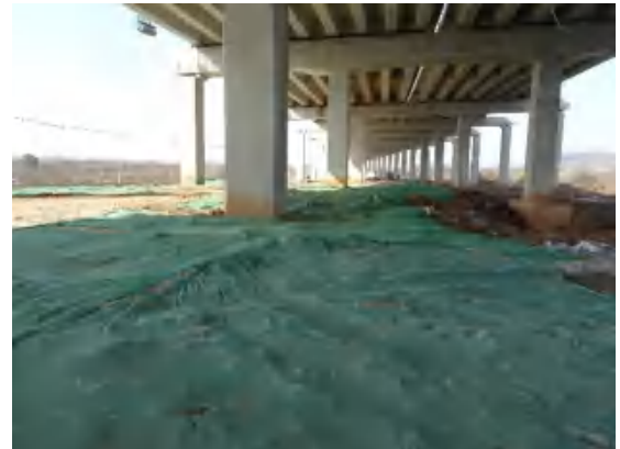
K9+800 桥下迹地防护网苫盖
