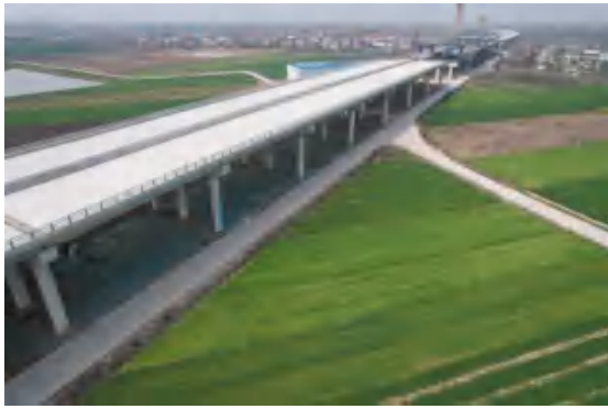
K30+500 桥下防护网苫盖
