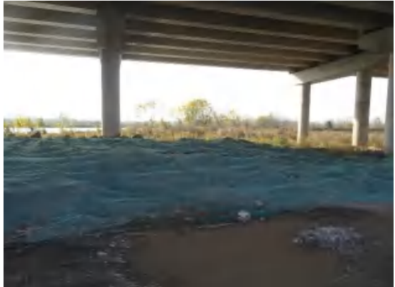
K31+100 桥下防护网苫盖
