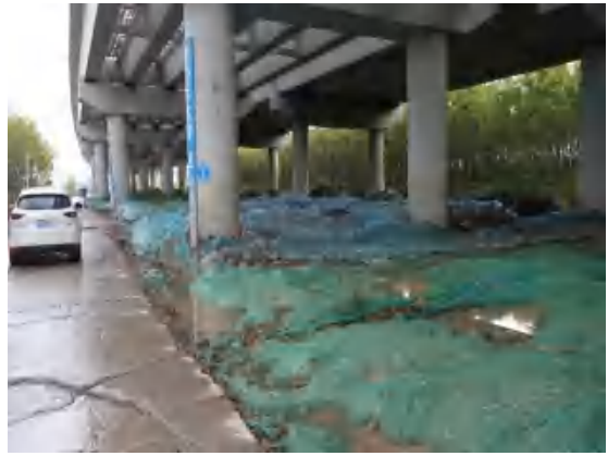
K29+300 桥下迹地防护网苫盖
